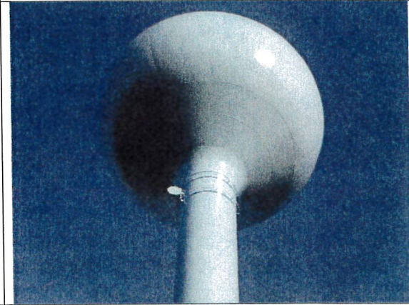
Exterior view of finish coat.
