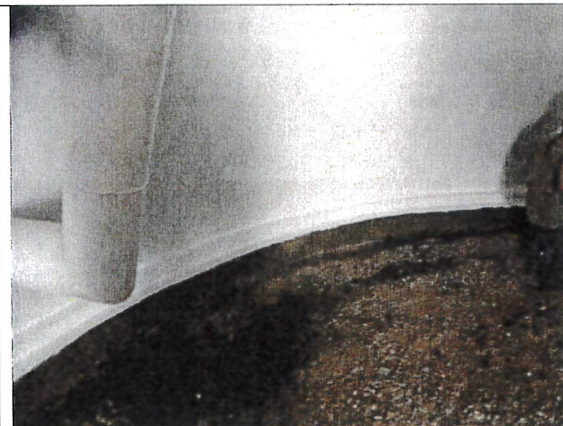
Tops of concrete foundation painted tank white.
