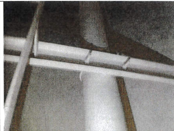
Dry interior pedestal second coat.
