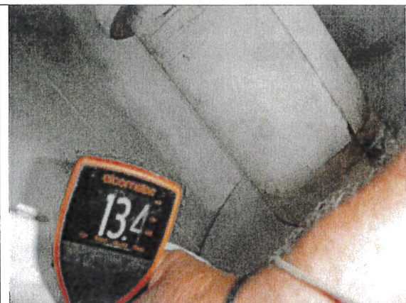
Dry interior second platform second coat.
