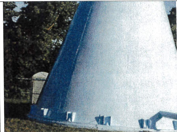
Exterior view of finish coat.
