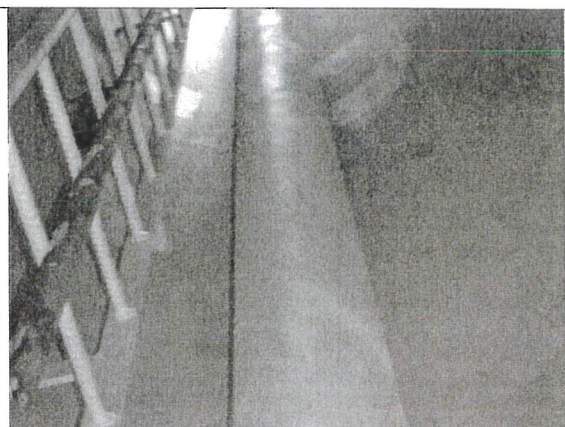
Dry interior access tube second coat.
