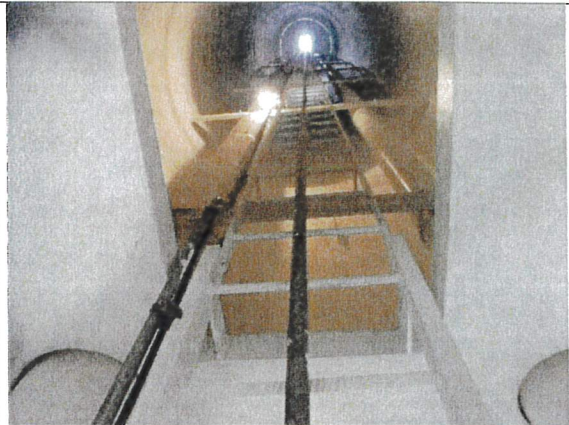
Spot repairs dry interior condensation platform.
