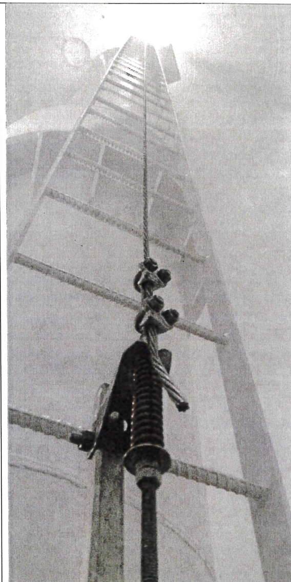
Wet interior fall prevention in place.
