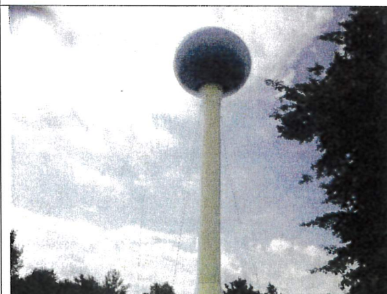
Exterior view tank.
