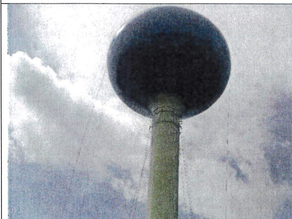
Exterior view tank.
