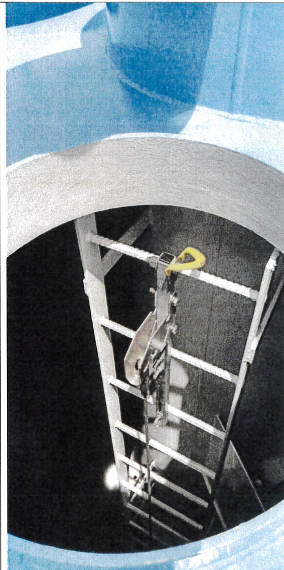
Wet interior fall prevention in place.
