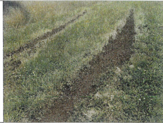
Filling of ruts in lawn completed.
