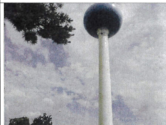
Exterior view tank.
