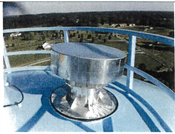
Exterior roof vent.
