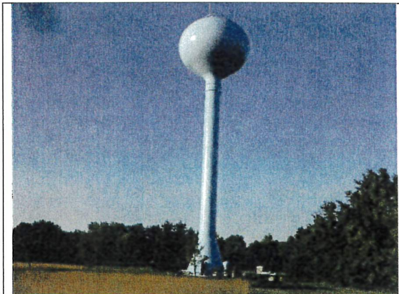
Exterior view of finish coat.
