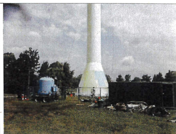
Exterior view tank.
