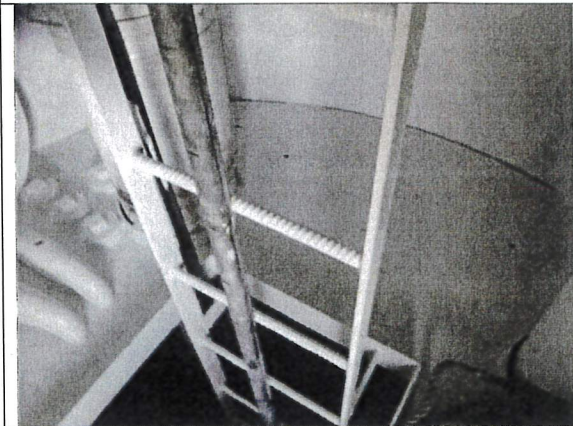
Ladder rungs received finish coat Tnemec tank white
